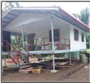
Construction of Poroi 2 Aid Post
