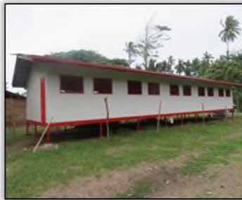
Construction of a double classroom for Arehava-Harevavo P/S, Larihairu Village.
